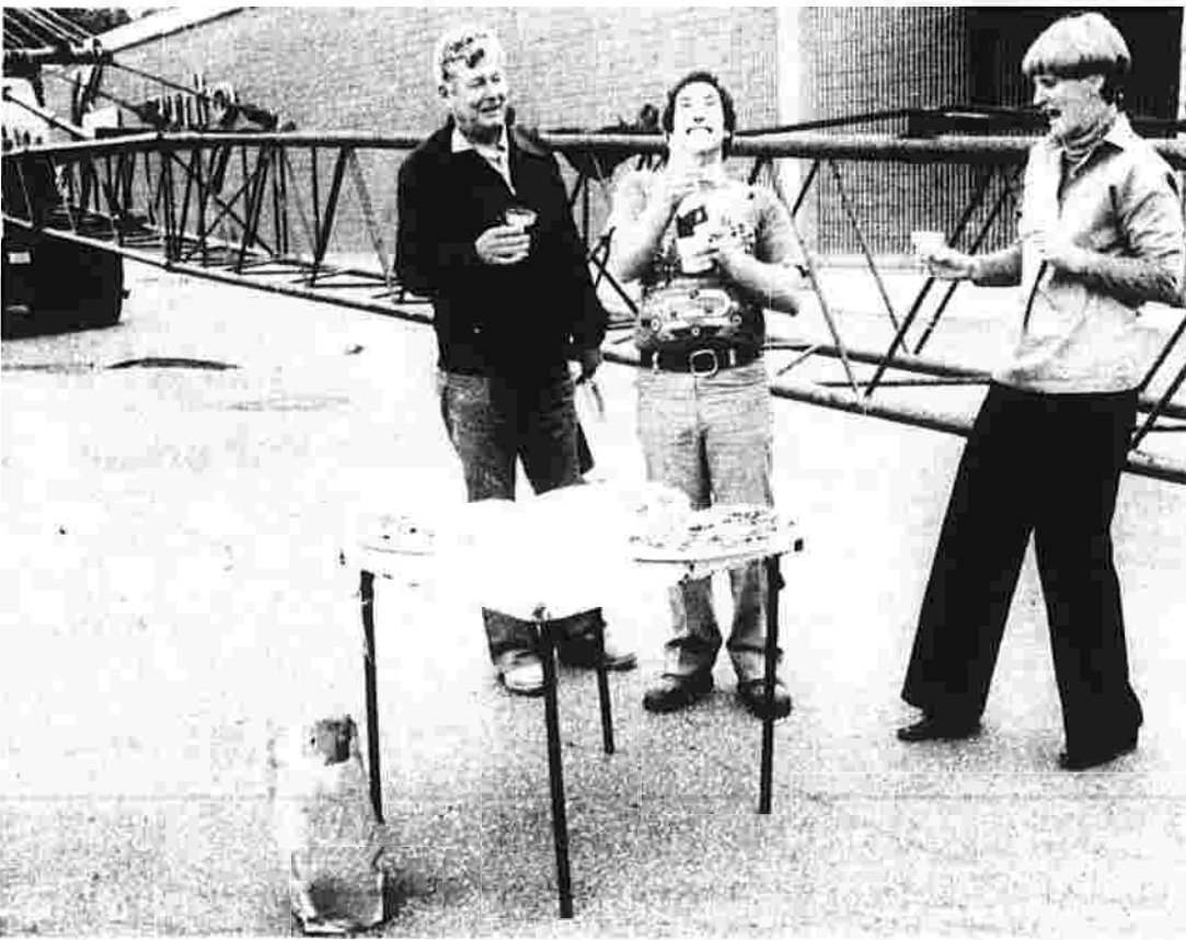
Tony LoGrasso, owner of the Pizza Wagon, brought out the champagne Friday afternoon to celebrate the start of reconstruction of the K-Mart where the roof collapsed under heavy ice and snow in January. (Herald photo by Strempler)
